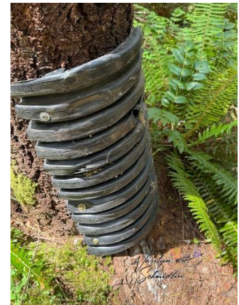
Well-worn culvert section in place with screws and washers
