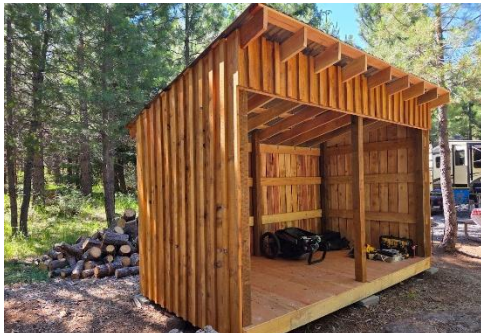
New shed on our southern property
