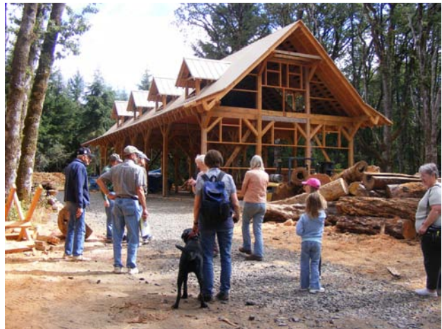
The barn being built at Zena Woods is a tribute to the family's German heritage using timber construction with mortise and wooden peg joints
